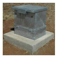
Internal heating is provided in cold climates where condensation is a problem. The following picture serves as illustration:
